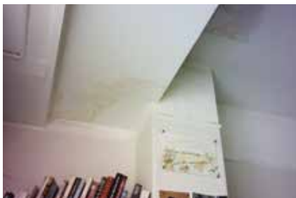
Hot water pipes hidden behind the wall are leaking. In this case visual signs of water leakage are present. The thermal imaging camera helps to pinpoint the leak location.
