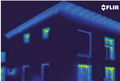
Thermal image shows insulation quality of a low energy house.
