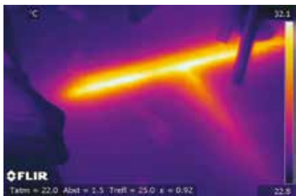
This thermal image shows where the hot water pipe has been installed beneath the floor.
