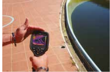
The FLIR thermal imaging camera clearly localized the water leaks.
